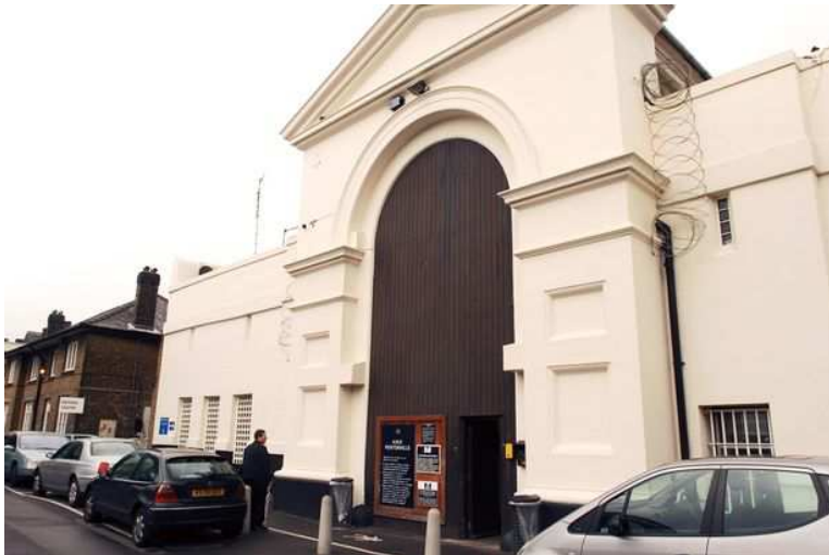
HMP Pentonville in North London
