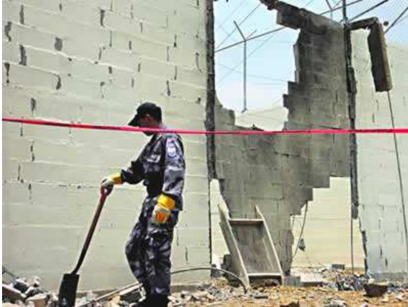
Destroyed walls of "La Roca"
